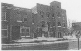
Photo 2 - 1910 Addition, South of Original Building
