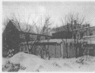
Photo 4 - 1957 Single Storey Addition
