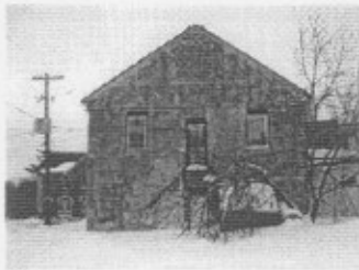
Photo 3 - 1873 Addition (Along Mill Street)
