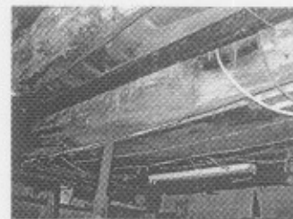
Photo 8 - Notched Hewn Log
