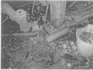
Photo 9 – Unfounded Wood Column
