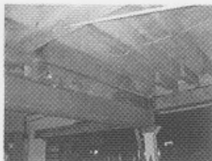
Photo 21 – Load bearing Wall Removal – 1910 Addition
