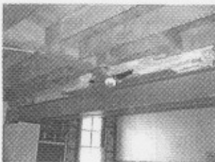
Photo 22 – Load bearing Wall Removal – 1910 Addition
