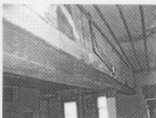
Photo 23 – Load bearing Wall Removal – 1910 Addition
