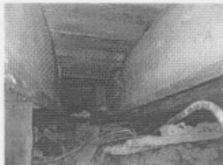
Photo 33 – Crawl Space (1980 Addition)
