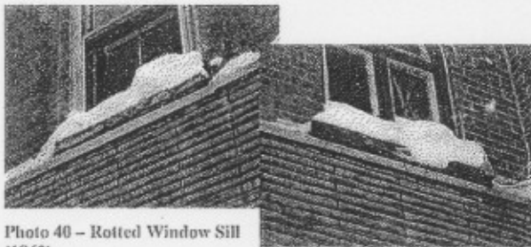
Photo 41 – Rotted Window Sill (1957)
